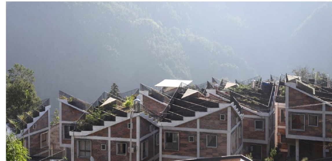
Reconstruction of Jintai Village located near Guangyuan, Sichuan Province — one of the places hardest hit by the May 12th Wenchuan Earthquake in 2008
